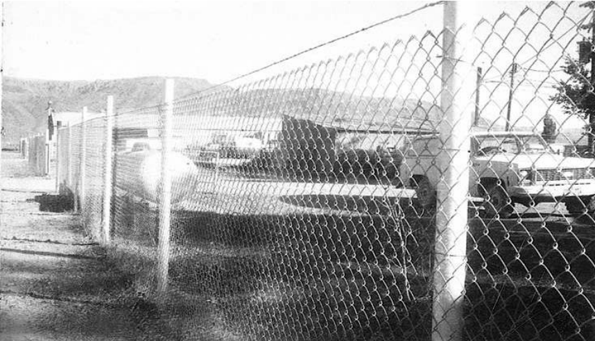
5' CHAIN LINK FENCE NO TOP RAIL
